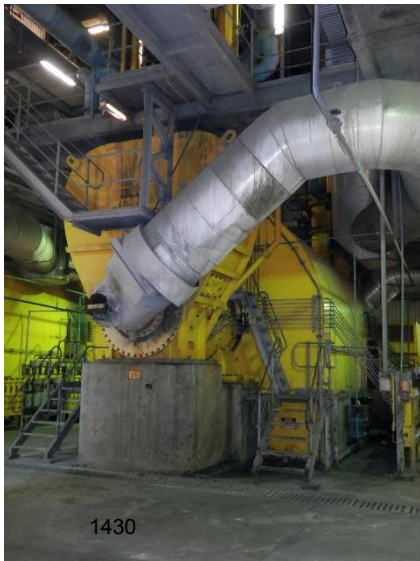
Coal Pulveriser
