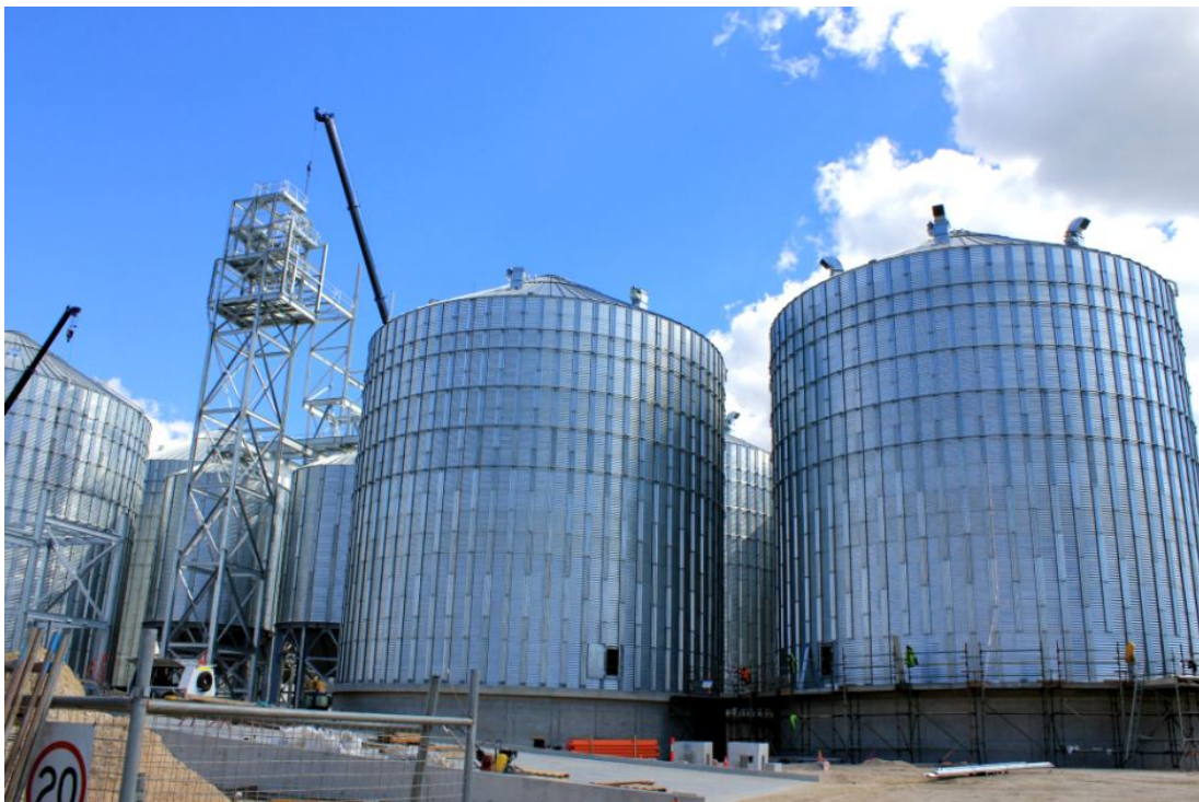
Figure 7 - Bunge Bunbury Grain Silos
