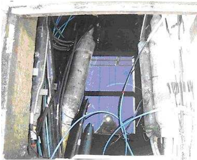
MANHOLE NEAR CNR FERNTREE GULLY RD & LUM RD, WHEELERS HILL (27-SEP-2001) NOTE COPPER CABLE JOINT ENCLOSURES AND NUMEROUS SMALLER SIZE CABLES (REFLECTION OF SKY/PHOTOGRAPHER IN WATER AT BOTTOM)
