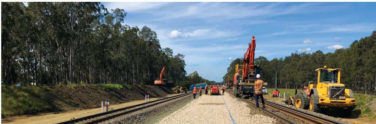
Photo: Hunter Valley AWP project worksite
