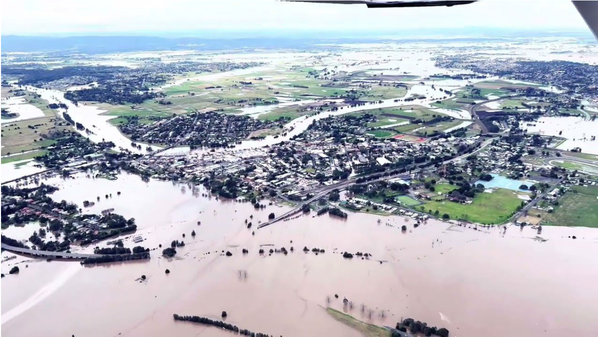
Figure 3: Flooding through Maitland 1
