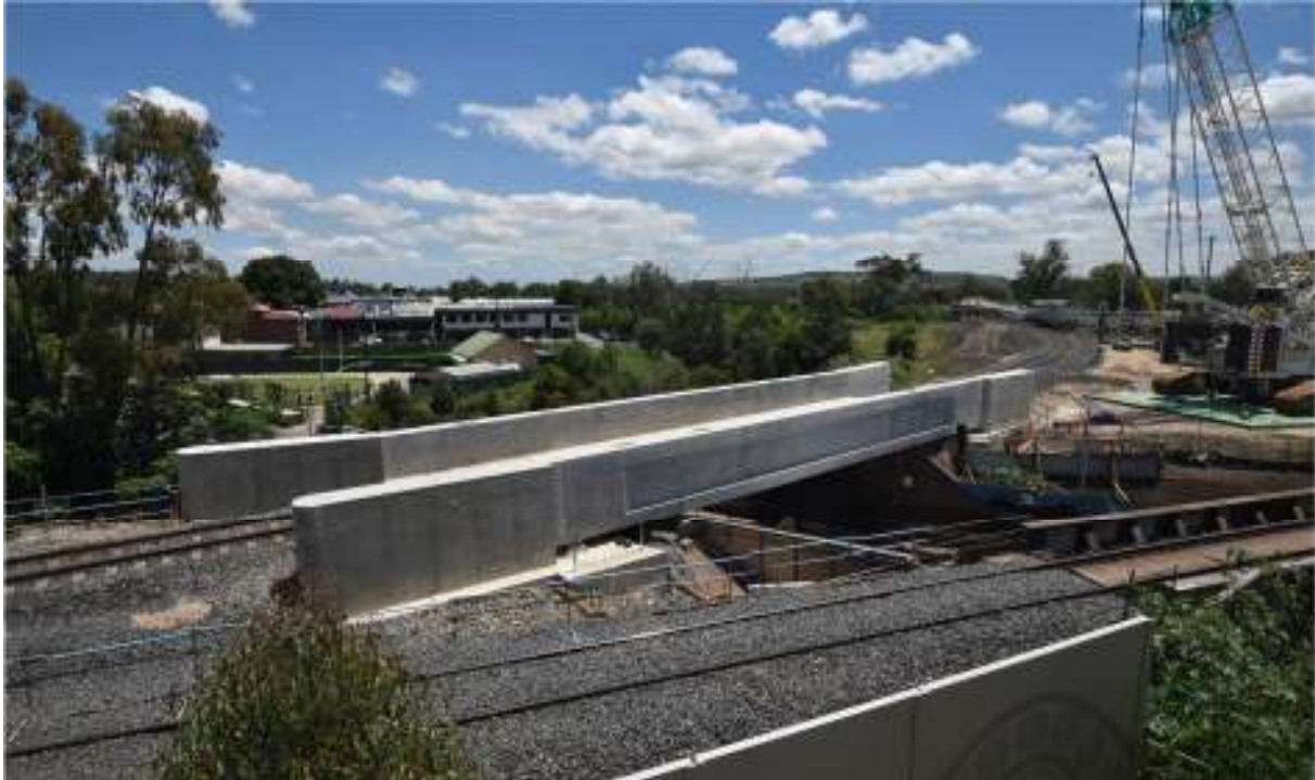
Figure 3: Construction work on the commissioned Bridge Street Bridge, Muswellbrook.
