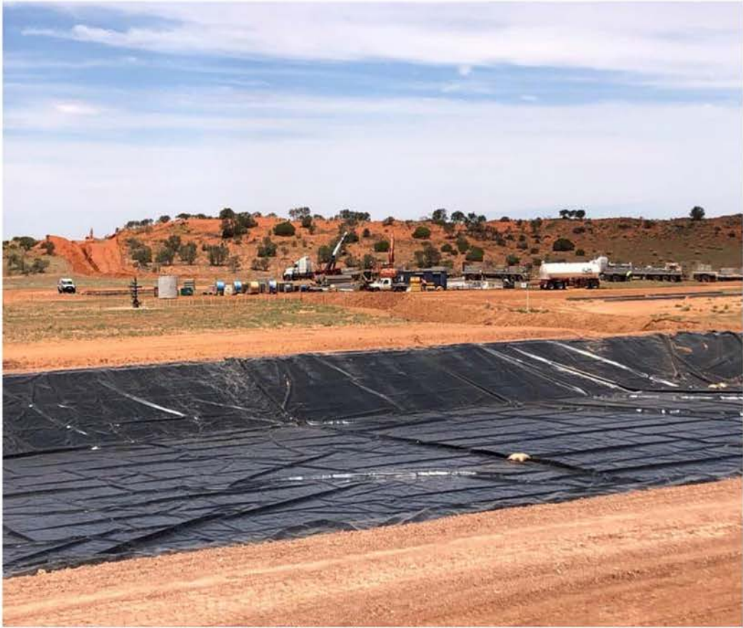
Installed pond liner with Vali-1 well site and laydown area
