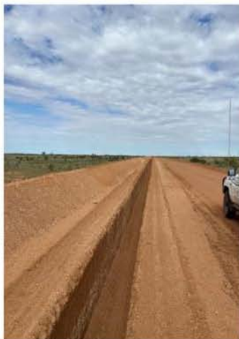
Completed trenching for installation of Fibrespar export line
