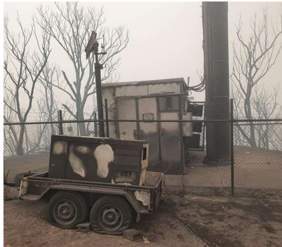
Figure 5. Jingellic mobile and radio tower with portable generator at front, following the Black Summer bushfires
